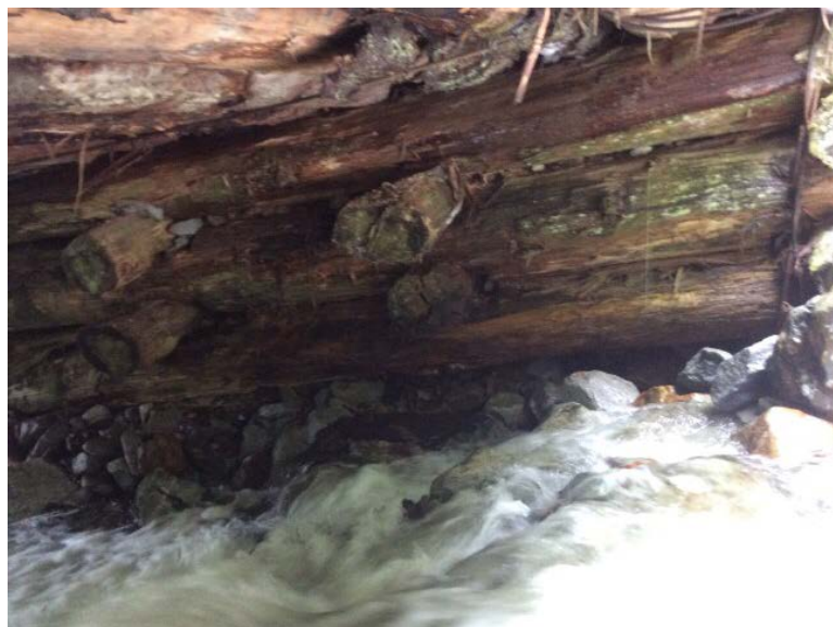
Right Bank Abutment when facing downstream
